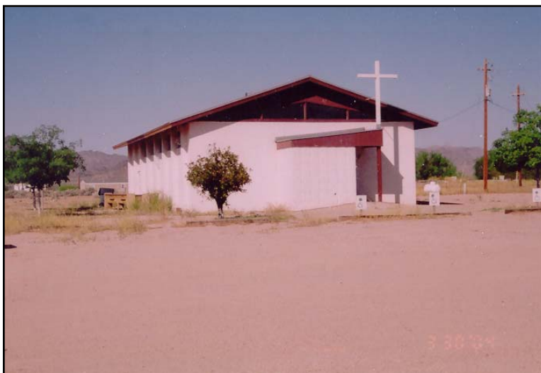
Figure 2: District Six Gila Crossing Presbyterian Church, Main Entrance (before and after exterior remediation)
