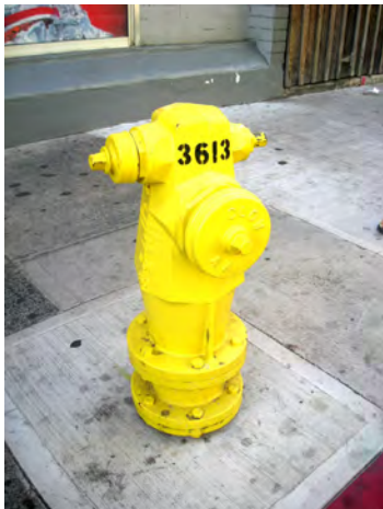
Figure 4.6. A wet barrel fire hydrant. The operating nut for the small hose outlet is on the right. The operating nut for the large outlet is on the rear of the hydrant.
