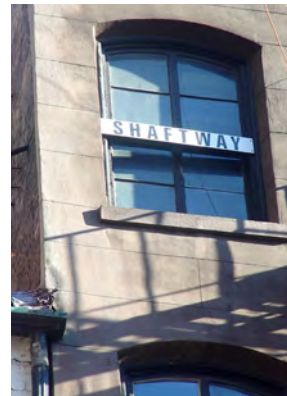
Figure 7.10. Exterior shaftway marking.
