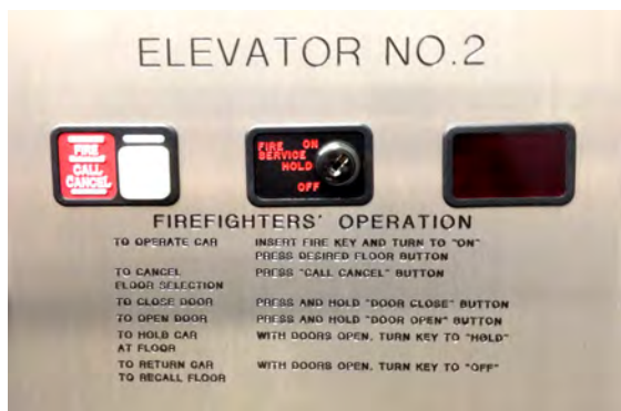
Figure 6.12. Elevator cab controls for Phase 2 firefighter operation.
