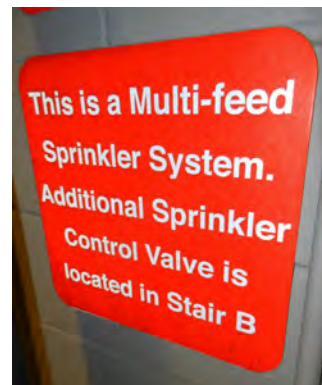
Figure 8.8. A sign near a sprinkler control valve indicating the location of the other valve that controls the same system.
