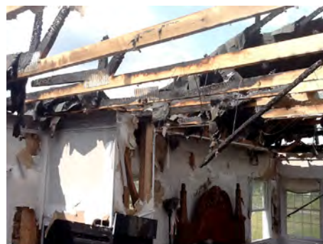
Figure 7.8. Wood trusses after an attic fire.
