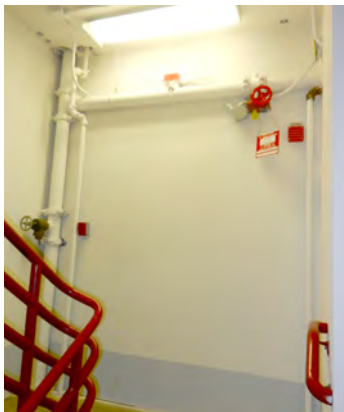
Figure 9.19. A standpipe isolation valve on a feed main (entering horizontally from the upper right) leading to a vertical standpipe riser (on the left). The valve is located within the stair enclosure to protect both the valve and the firefighters who may need to access it.
