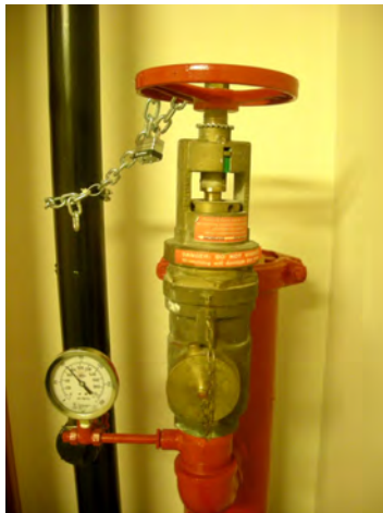
Figure 9.6. An FHC equipped with a pressure-regulating device.
