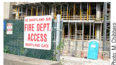
Figure 13.5. Temporary fire apparatus access.
