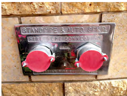
Figure 10.3. A combined sprinkler and standpipe FDC.
