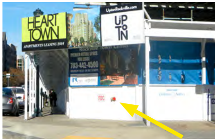
Figure 13.6. A temporary FDC (see arrow) feeding a standpipe being installed as this building rises.
