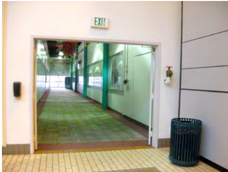
Figure 9.10. A double set of horizontal exit doors. One FHC is shown to the right of the doors; another is on the opposite side.
