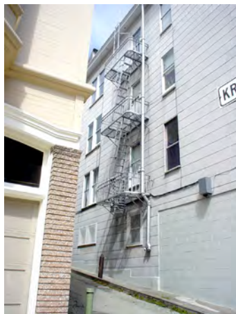
Figure 9.1. An exterior dry standpipe with an FDC on the bottom and a FHC at each fire escape platform.
